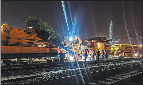
Employees from Taiyuan North Railway Station in Shanxi province work on phase-II of the concentrated overhaul of the Shijiazhuang-Taiyuan Railway. China Railway Taiyuan Group launched the move in a bid to ensure safer rail transport.
