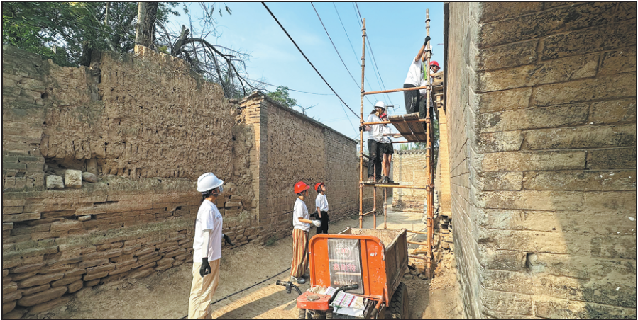
From left: Workshop members line up to convey bricks at the renovation site in Dongquan village. Members peel off the solid mortar layers on bricks to be used in rebuilding walls in Dongquan.
