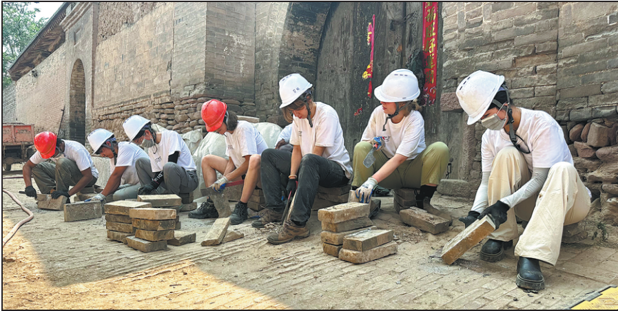
From left: Workshop members line up to convey bricks at the renovation site in Dongquan village. Members peel off the solid mortar layers on bricks to be used in rebuilding walls in Dongquan.
