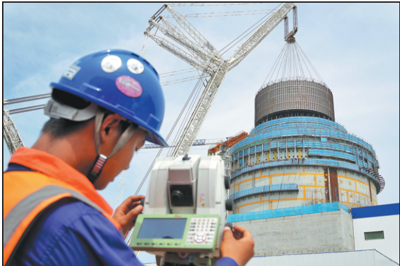
An engineer monitors the hoisting of a module of the No 3 generator set at Haiyang Nuclear Power Plant in Haiyang on Aug 4. TANG KE / FOR CHINA DAILY
