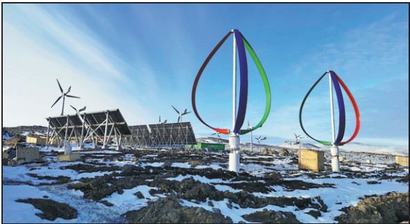
The water-drop-shaped devices are the latest wind turbine developed by Taiyuan University of Technology, which feature effective resistance to low temperatures and strong winds. PROVIDED BY TAIYUAN UNIVERSITY OF TECHNOLOGY
