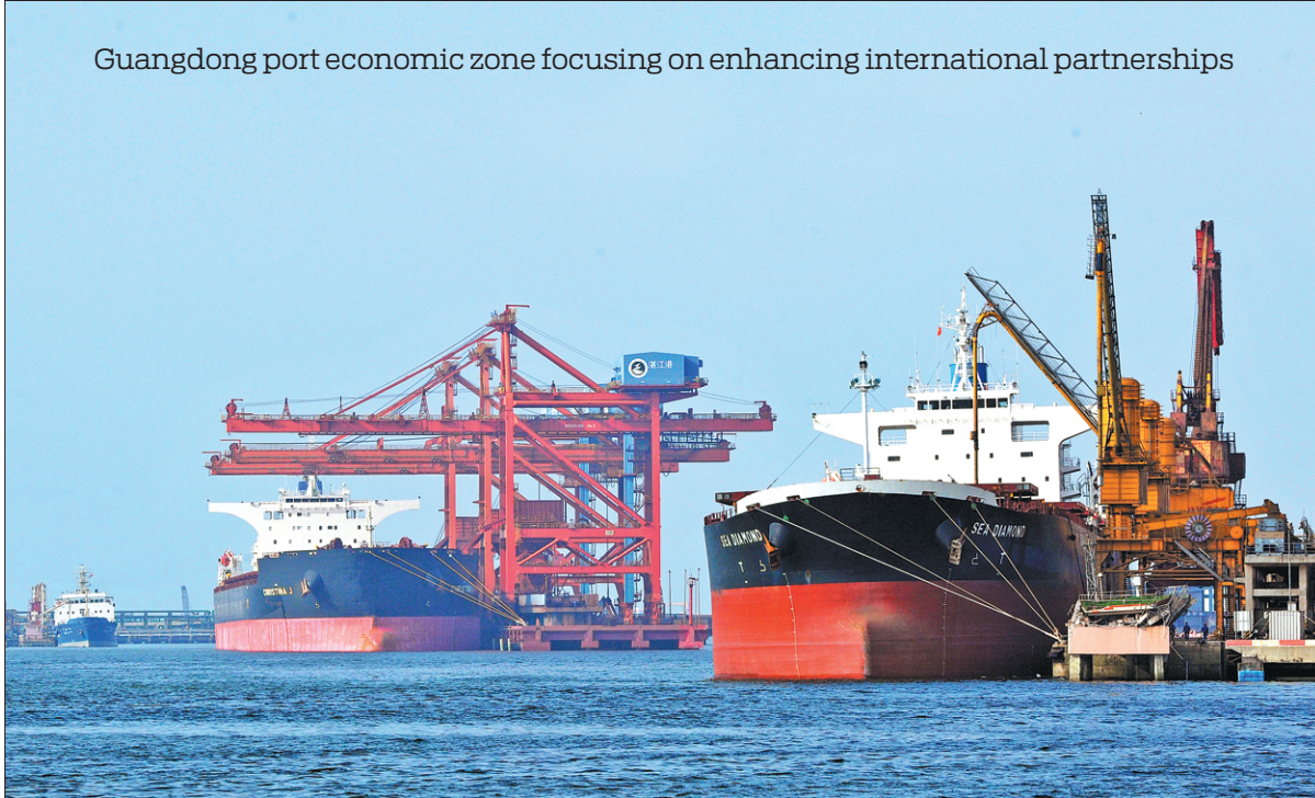
Zhanjiang Port, one of China's 25 main coastal ports, can handle 400,000-dead-weight tonnage ships. PHOTOS PROVIDED TO CHINA DAILY
