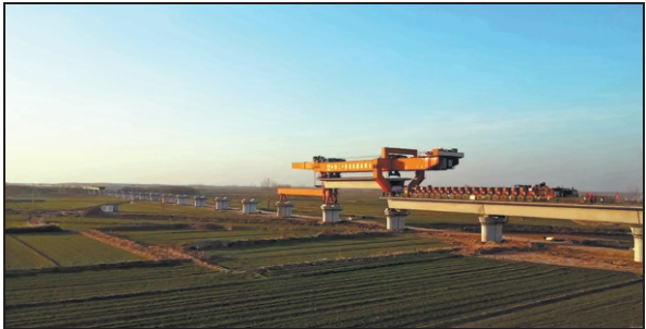
A drone image shows the installation of a box girder on the Jinan-Binzhou High-speed Railway in Binzhou, Shandong province. The 145-kilometer-long HSR, featuring an operating speed of 350 km per hour, is the first HSR to link downtown Binzhou with the provincial HSR network, said China Railway Construction Corp's 24th bureau, a State builder involved in the project. PROVIDED TO CHINA DAILY
