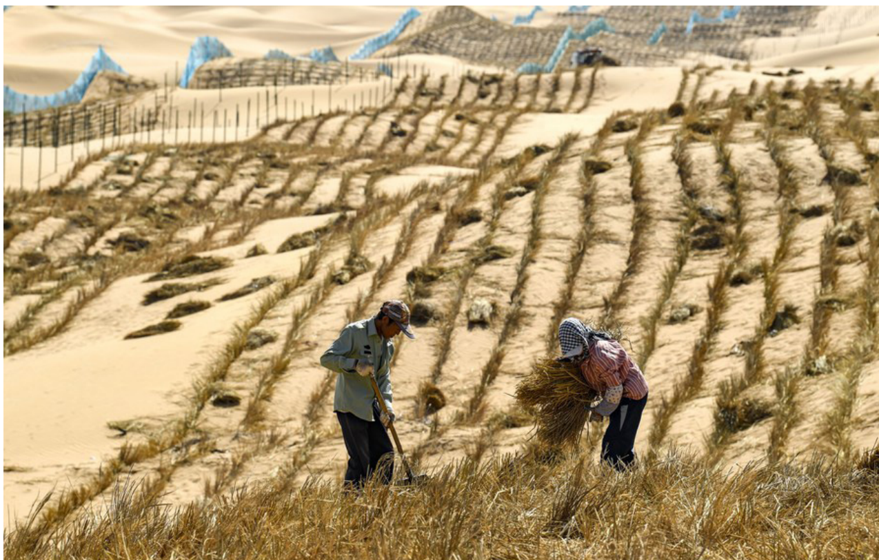
File photo taken on September 7, 2020 shows desertification control workers making straw-checkerboard barriers in the Tengger Desert, along the construction site of the Qingtongxia-Zhongwei section of the Wuhai-Maqin highway in Northwest China's Ningxia Hui Autonomous Region. [IMAGE: XINHUA/FENG KAIHUA]
