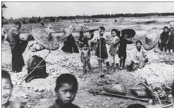
Children from Sichuan province participated in building the airport runways for the US air force from 1937 to 1943.
