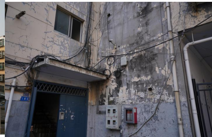
Peeling Exterior Walls
