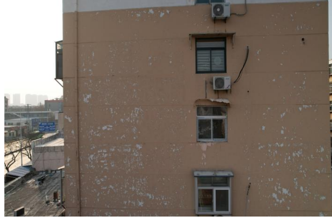
Peeling Exterior Walls
