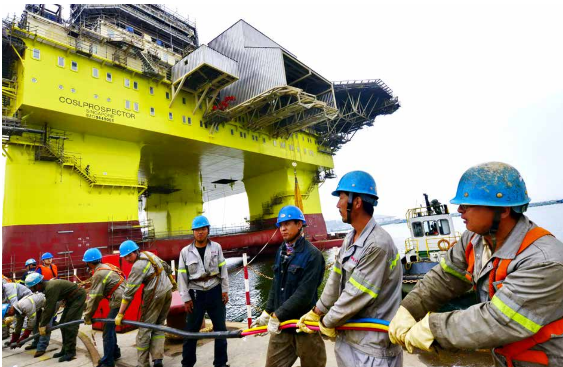
正在建造中的海上石油钻井平台 An offshore oil-drilling platform being built
