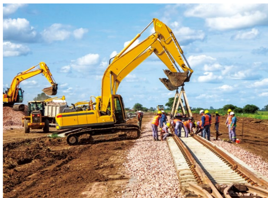
◆ Belgrano freight railway reconstruction project undertaken by CMEC
