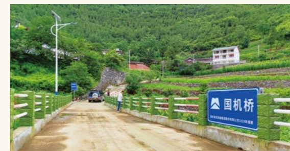
◆ SINOMACH Bridge in Chaotian District, Guangyuan City, Sichuan Province
