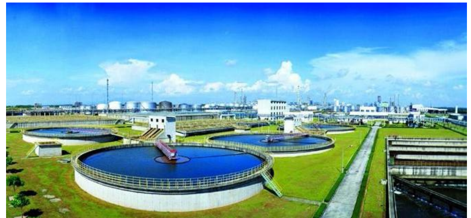
The ethylene effluent disposal plant owned by Sinopec Maoming Petrochemical Company
