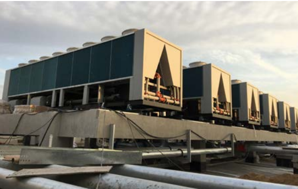
Installation site of the air-cooled chiller for the computer room of Tiandulu Data Center of the Anhui Branch in January 2020
