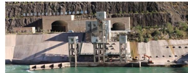
Fish Lifting Facility at Huangdeng Hydropower Station
