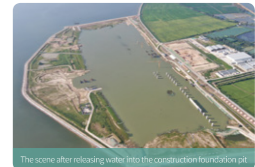
The scene after releasing water into the construction foundation pit
