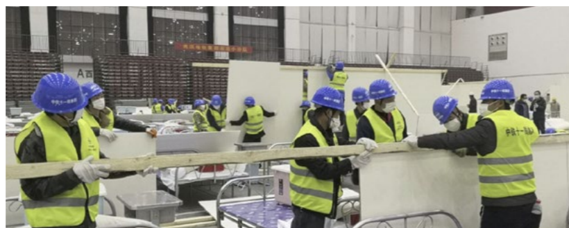
● 抢建武汉客厅“方舱医院” Rushing to build "mobile cabin hospitals" in Wuhan
