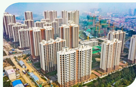
◆ 打造高品质安置房 Building high quality resettlement housing
