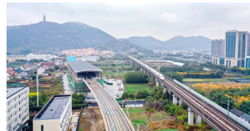
● 建设中的杭绍城际铁路 Hangzhou-Shaoxing Intercity railway under construction
