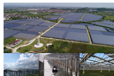
CECEP (Changxing) PV-Energy Storage Demonstration Project
