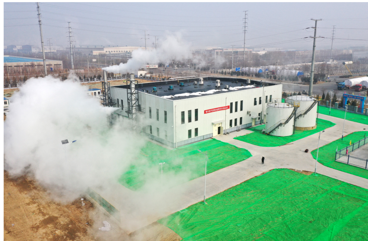
Digital integrated energy project at Yinchuan Economic and Technological Development Zone
