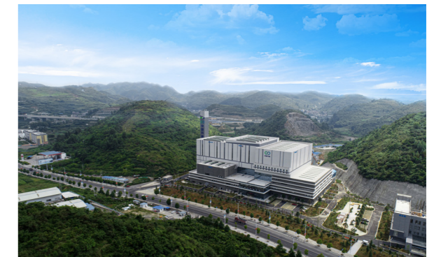
In July 2020, CECEP Bijie Comprehensive Solid Waste Treatment Industrial Park was officially put into operation.
