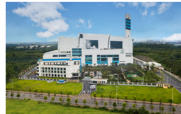
In April 2020, the household waste incineration power generation project in Jintang, Chengdu, Sichuan Province was officially put into operation.
