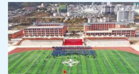
On November 26, CCCG's "turnkey" project Lanping New Era Hope School was officially completed
