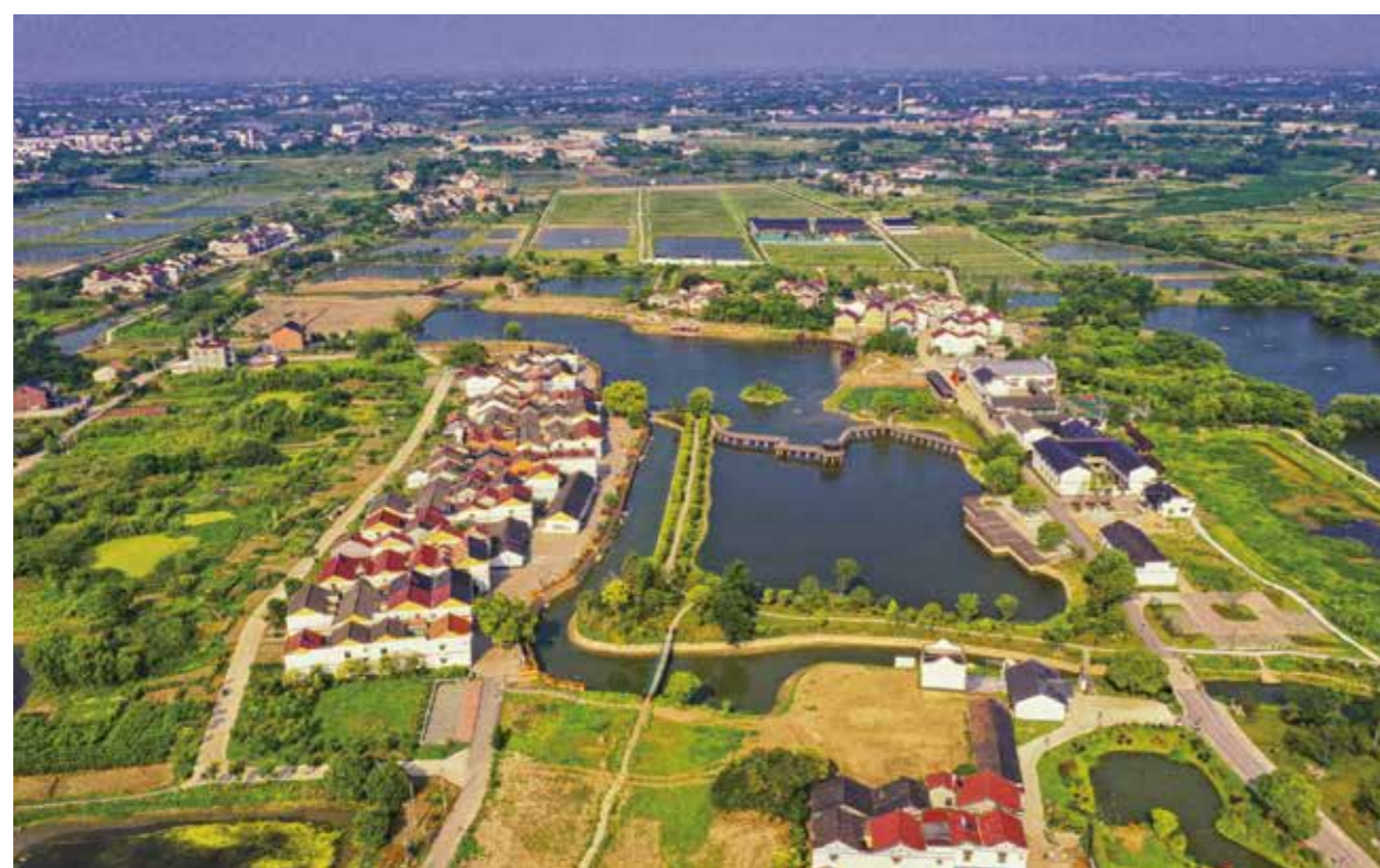
Project Baiyang Qianhe at Huzhou
