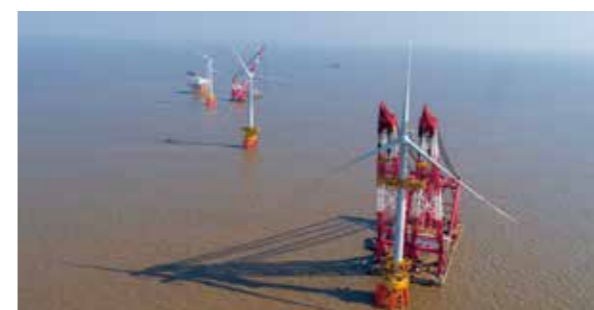
Guodian Offshore Wind Farm 6 Zone 2 in Putuo District of Zhoushan
