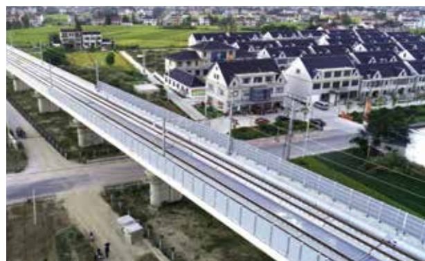
Trial operation of the Yancheng-Nantong High-speed Railway in Jiangsu Province, an important part of the "coastal passage"
