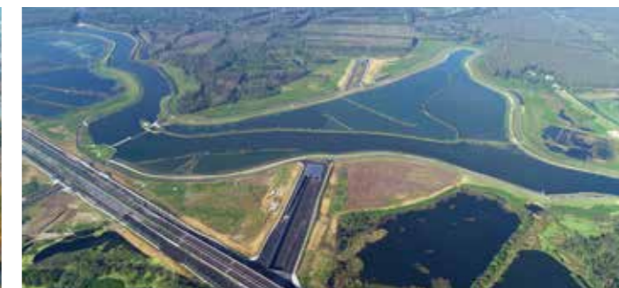
Ecological treatment project of wetland water quality in the Lower Reaches of Shibuli River in Anhui
