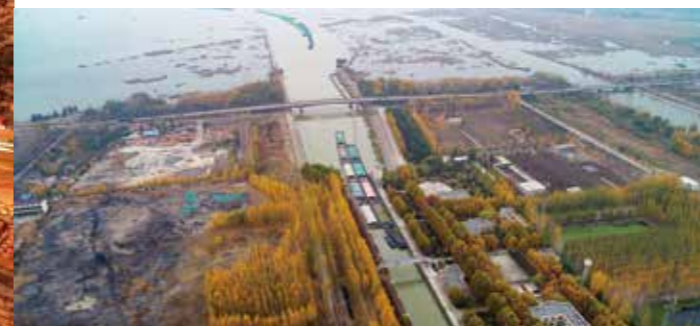
Treatment project of waterway of Beijing-Hangzhou Grand Canal in Shandong
