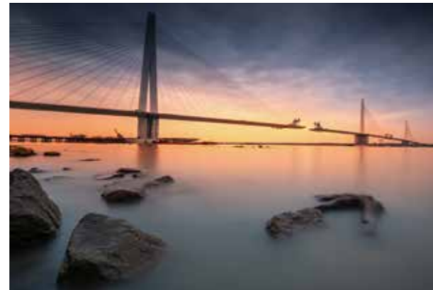
Nanjing Jiangxinzhou Yangtze River Bridge (Nanjing Yangtze River Fifth Bridge) is completed and opened to traffic
