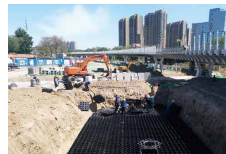
Installation of PP reservoir modules
