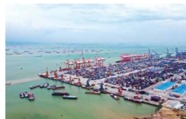
With the deep-water channel widening project put into operation, the Guangzhou Port has officially entered a new "two-lane" era
