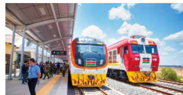
Mombasa-Nairobi Standard Gauge Railway, Kenya
