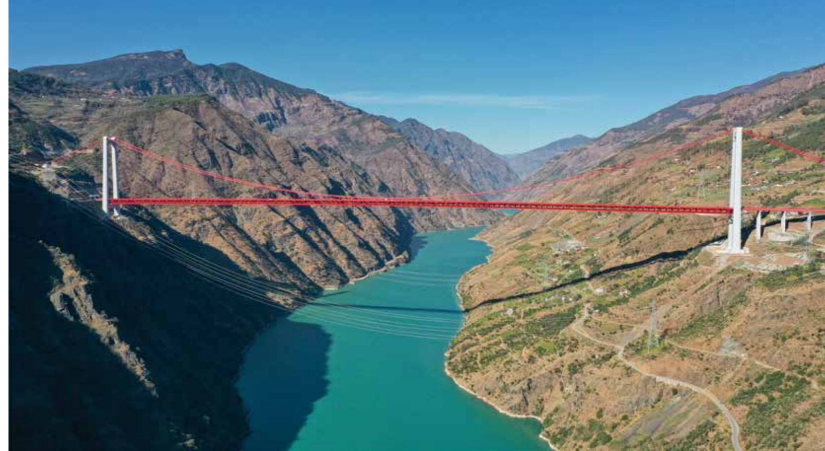
Panoramic view of the Jin'an Jinsha River Bridge of Huaping-Lijiang Highway
