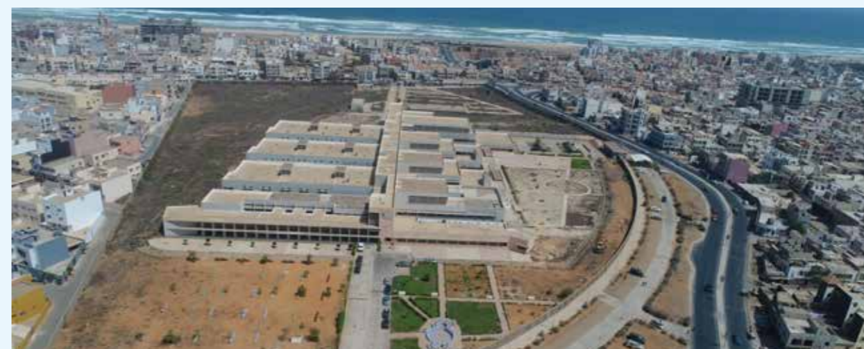
CRBC assists in the construction of Senegal's "Huoshenshan" Hospital for free
