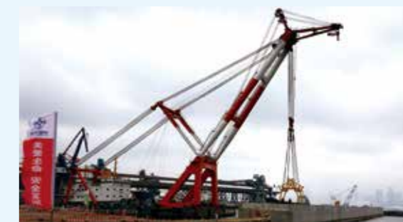
On February 28, Dalian Bay Subsea Tunnel Project resumed work and production
