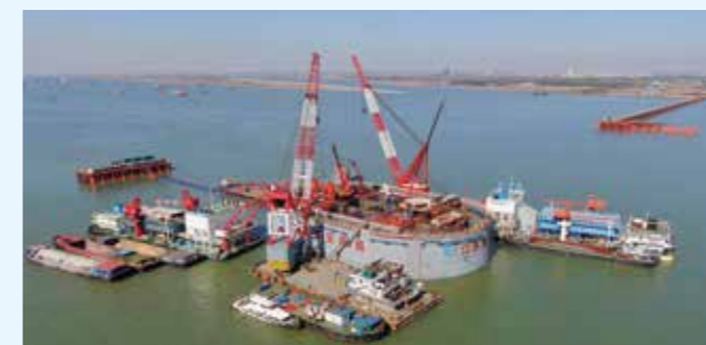
On February 18, the world's largest-span road-rail steel truss cable-stayed bridge was built with the participation of CCCG Second Harbour Engineering—The sandwich wall concrete of the steel caisson of the main bridge of Changtai Yangtze River Bridge began its pouring for the first time
