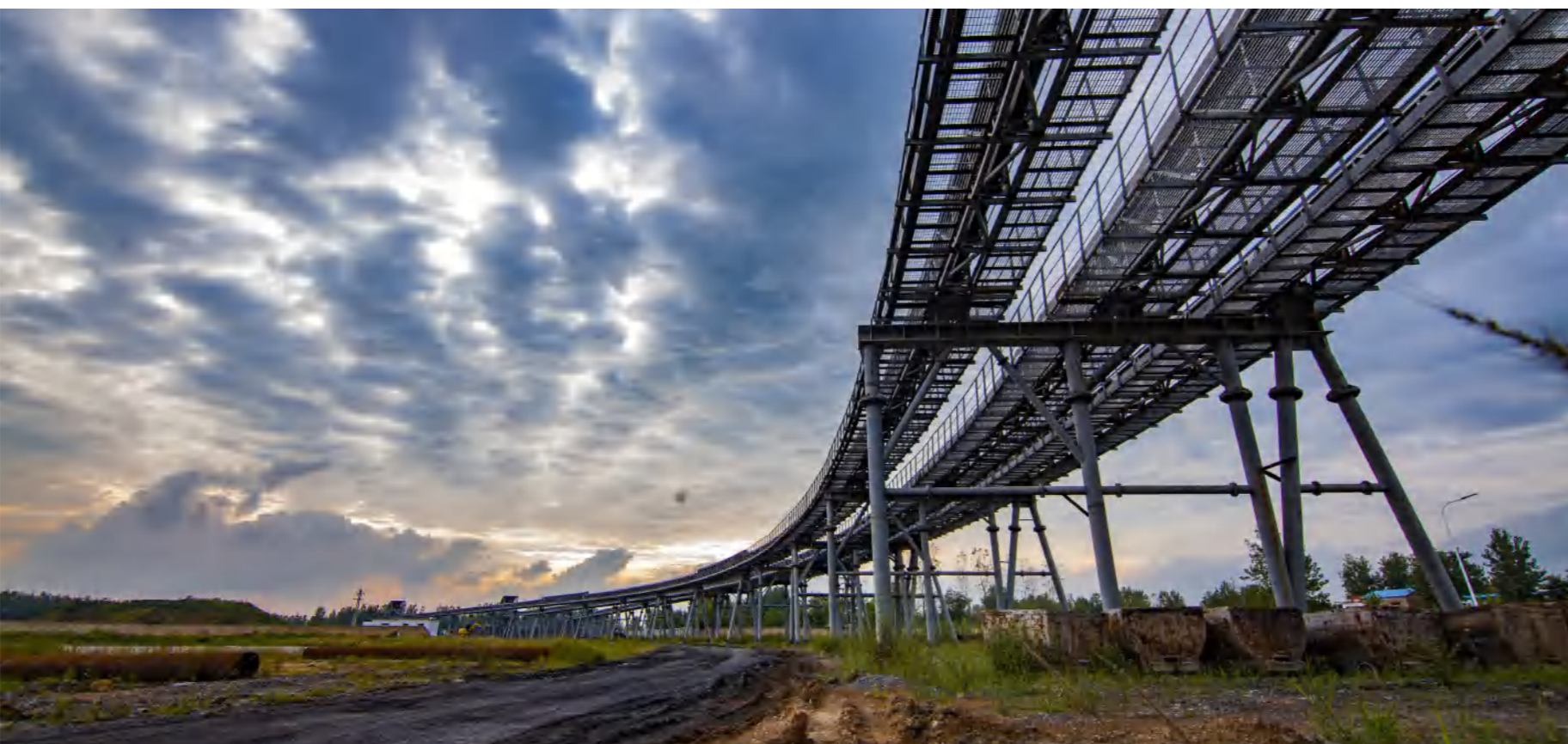
▲ DG250 pipe belt conveyor of Zhangzhuang Mine
