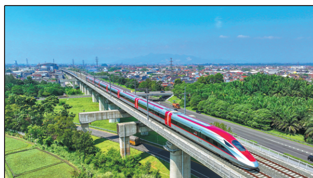
The Jakarta-Bandung High-Speed Railway is a flagship project of the Belt and Road Initiative cooperation between China and Indonesia. PROVIDED TO CHINA DAILY
