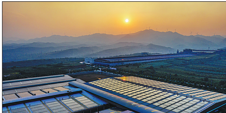
With photovoltaic panels installed on rooftops, a solar farm in Yuanqu county supplies clean power to local grids. XUE JUN / FOR CHINA DAILY
