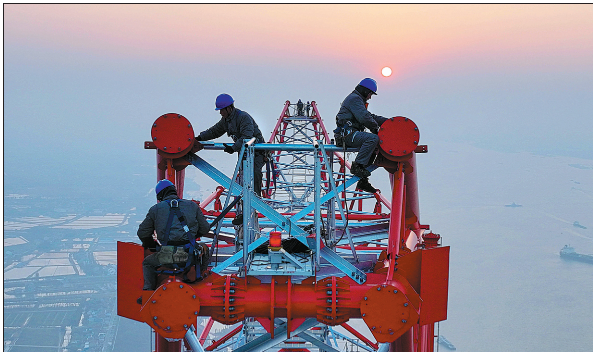
Construction workers complete the final part of a 385-meter power transmission tower in Taizhou, Jiangsu province, on Wednesday. The tower will help to transmit electricity across the Yangtze River between Fengcheng and Meili in Jiangsu to ease power shortages in those areas. TANG DEHONG / FOR CHINA DAILY
