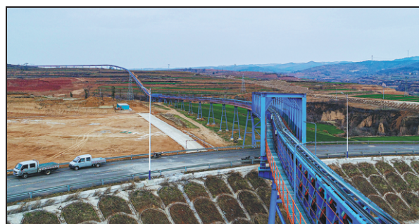
The 8.4-kilometer pipeline built by Huayu Coal Chemicals is the longest in Asia for coal transportation. JIAO ZHAOZHAO / FOR CHINA DAILY
