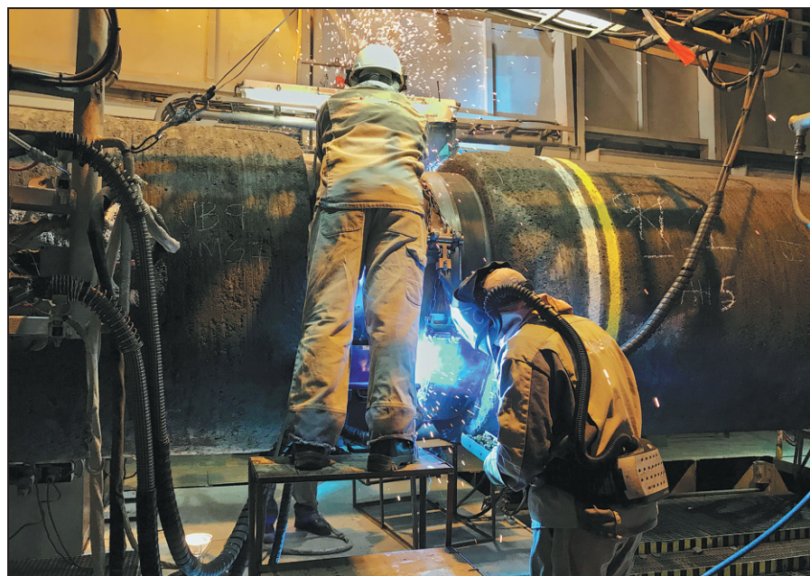
Specialists work onboard the deep sea pipe-laying ship Solitaire for the Nord Stream 2 pipeline in the Baltic Sea on Sept 13. STINE JACOBSEN / REUTERS
