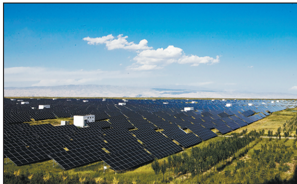
From left: A vast of photovoltaic panels work at a solar power farm in Qinghai. The province has rich resources in developing renewable energy. PROVIDED TO CHINA DAILY
