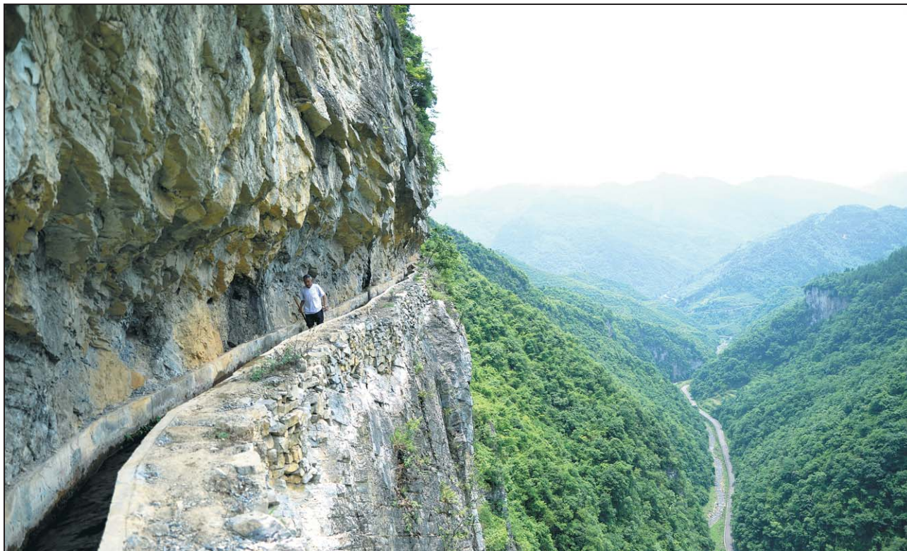
Irrigation channels are chiseled on the cliffs of mountains by Huang Dafa and his fellow villagers in Caowangba in Guizhou province's Zunyi. XING HAN / FOR CHINA DAILY
