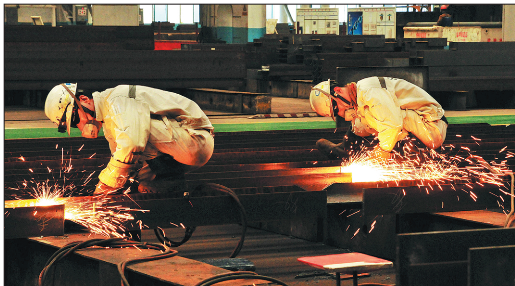
Workers cut steel plates at an offshore oil-drilling platform near Qingdao, Shandong province. YU FANGPING / FOR CHINA DAILY
