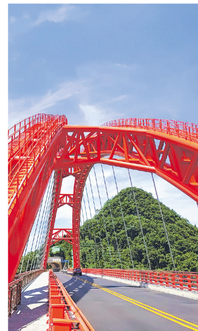
▲ The New Huayudong Bridge
