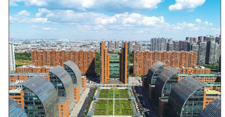
A financial center in the Tianjin Economic-Technological Development Area. PROVIDED TO CHINA DAILY
