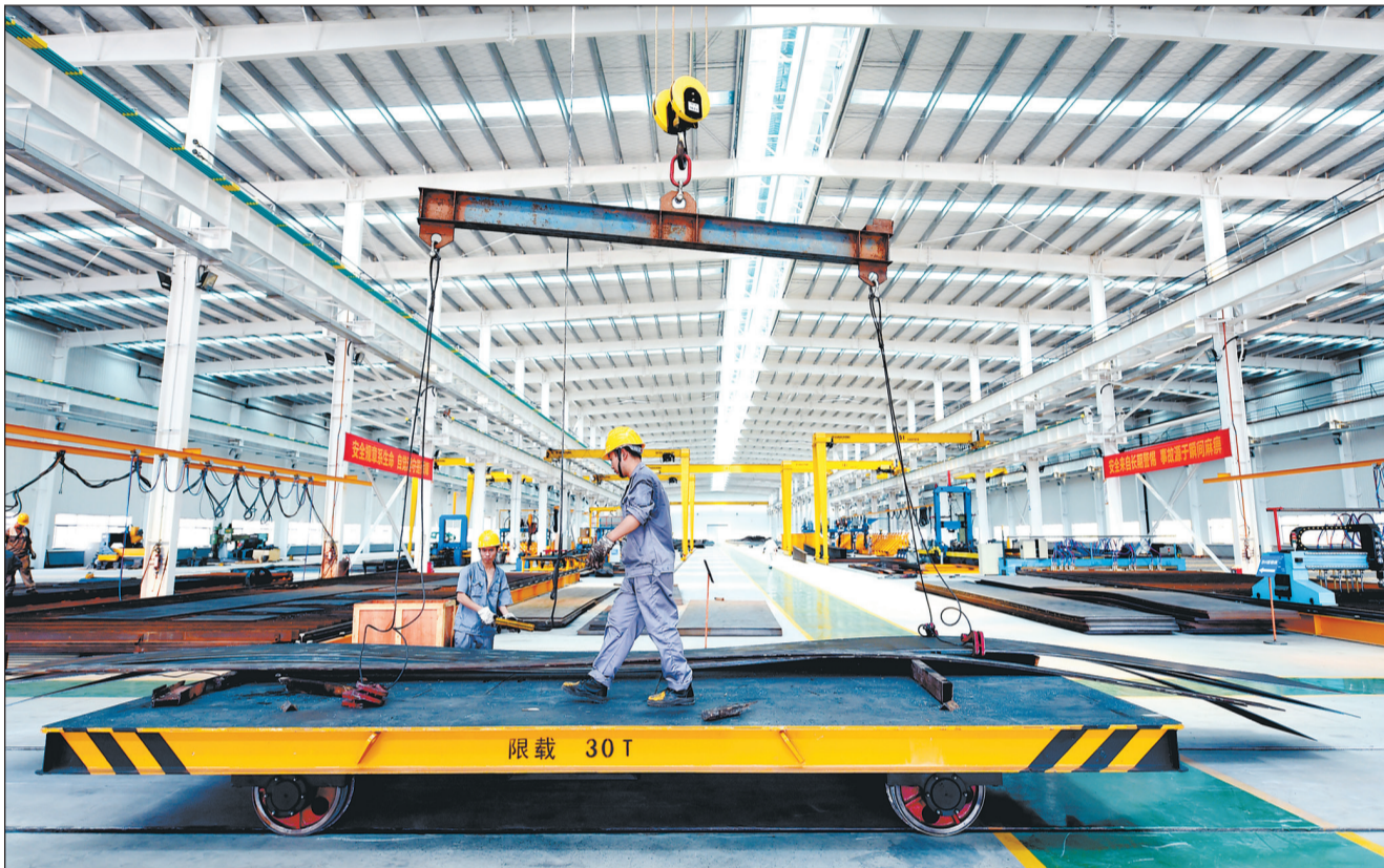
Zhanjiang Far East Steel Structure started trial production in early June and will export products to Indonesia in mid-July.
