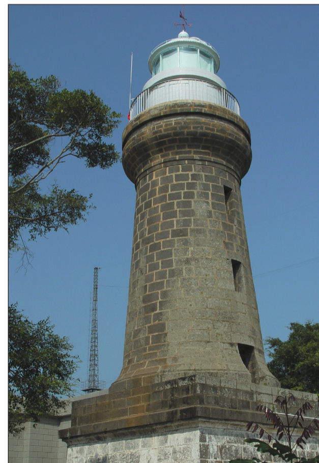
The Naozhou lighthouse, recognized as a cultural relic site under State-level protection, is a popular tourist attraction in Zhanjiang, Guangdong province. PROVIDED TO CHINA DAILY
