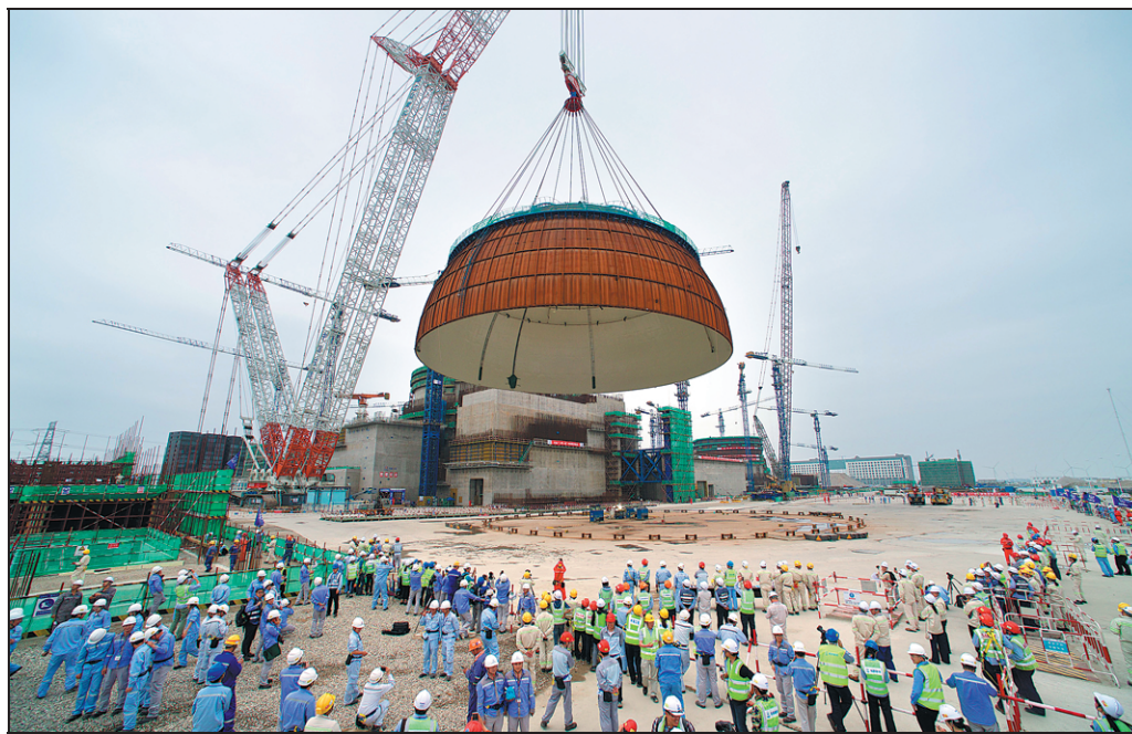
Builders install a dome on a fifth unit at the Hualong One Nuclear Power Station construction site in Fuqing, Fujian province, on Thursday. The next step is installing the unit’s equipment. The Hualong One uses third-generation nuclear power technology, which is developed and owned by China. JINAG KEHONG / XINHUA NEWS AGENCY
