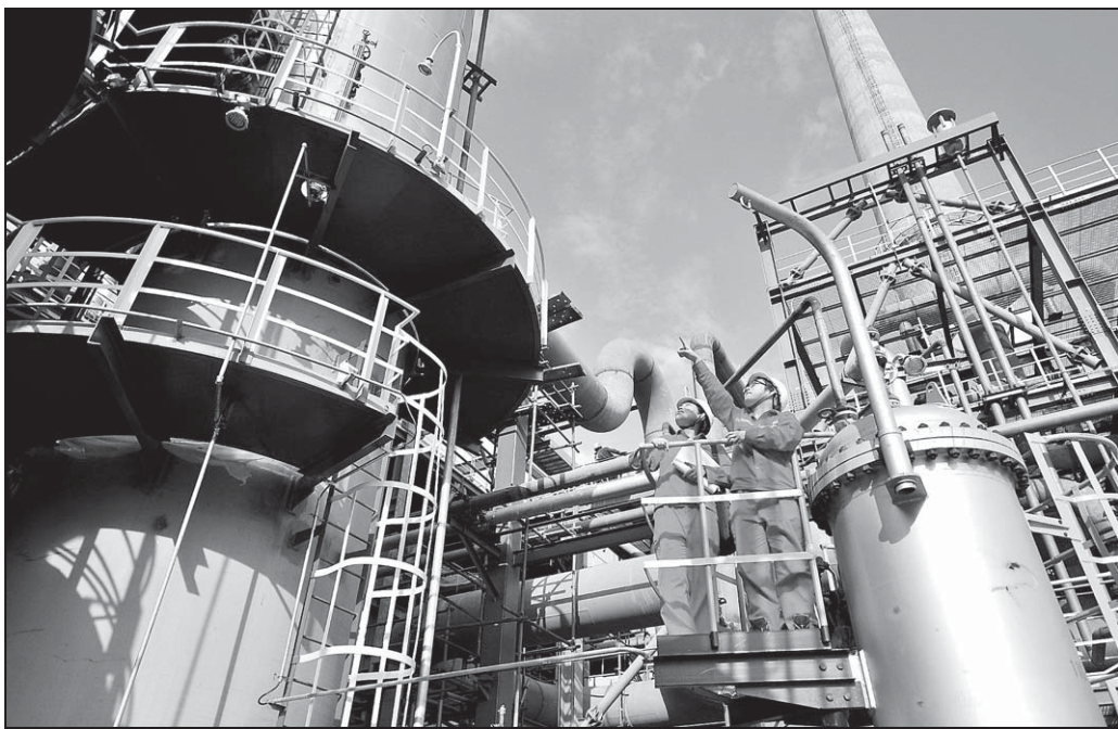
Sinopec employees check natural gas equipment in Guangyuan, Sichuan province, in June. HU QINGMING / FOR CHINA DAILY
