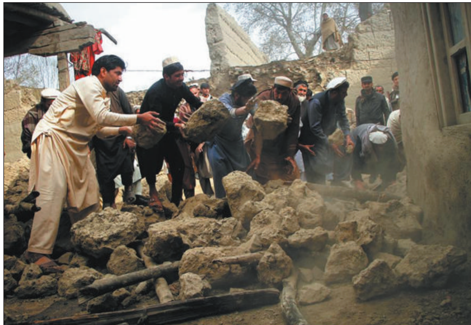
Local residents take part in rescue at the site of a house collapse in Nangarhar province, Afghanistan, on Monday. An Afghan woman and her four children were killed in the incident. XINHUA
