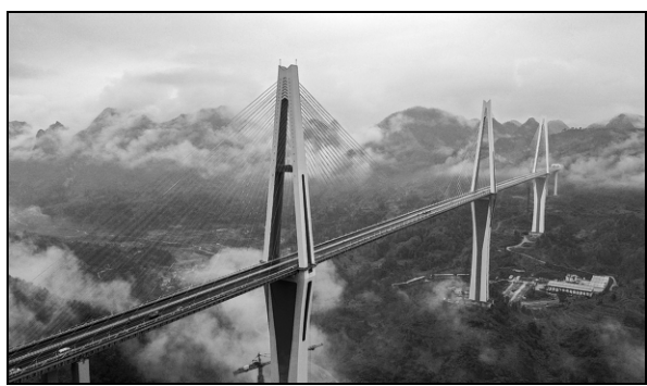
The Pingtang Grand Bridge in Guizhou province will open to traffic on Wednesday. YAN CHUNGUI / FOR CHINA DAILY
