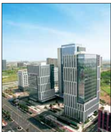
Nanjing Software Park is one of the high-tech engines in Jiangbei New Area. PROVIDED TO CHINA DAILY
