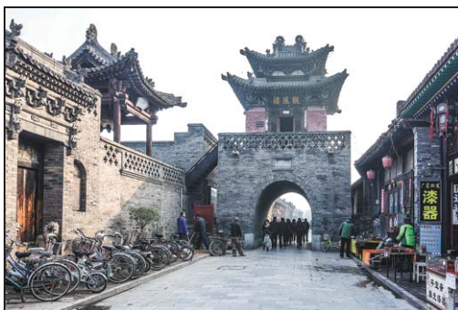
The Chinese city of Pingyao, built in the 14th century, is a UNESCO World Heritage Site for being an exceptionally well-preserved example of a traditional city. CHEN YAN / FOR CHINA DAILY
