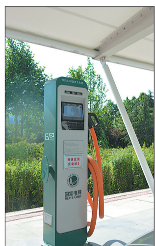
An electric-vehicle quick-recharging station in the Weifang High-Tech Development Zone.
