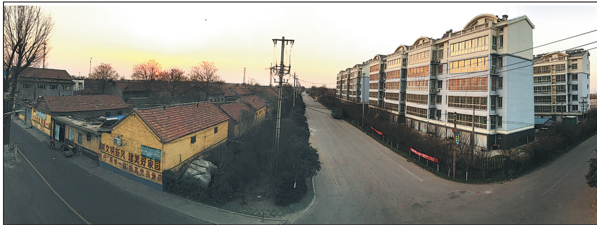
Top: Yuan Hengjun and his wife Yang Zhengxiang in their 112-square-meter apartment built in 2015 in Nanzhanglou village, Qingzhou city, Shandong province.
