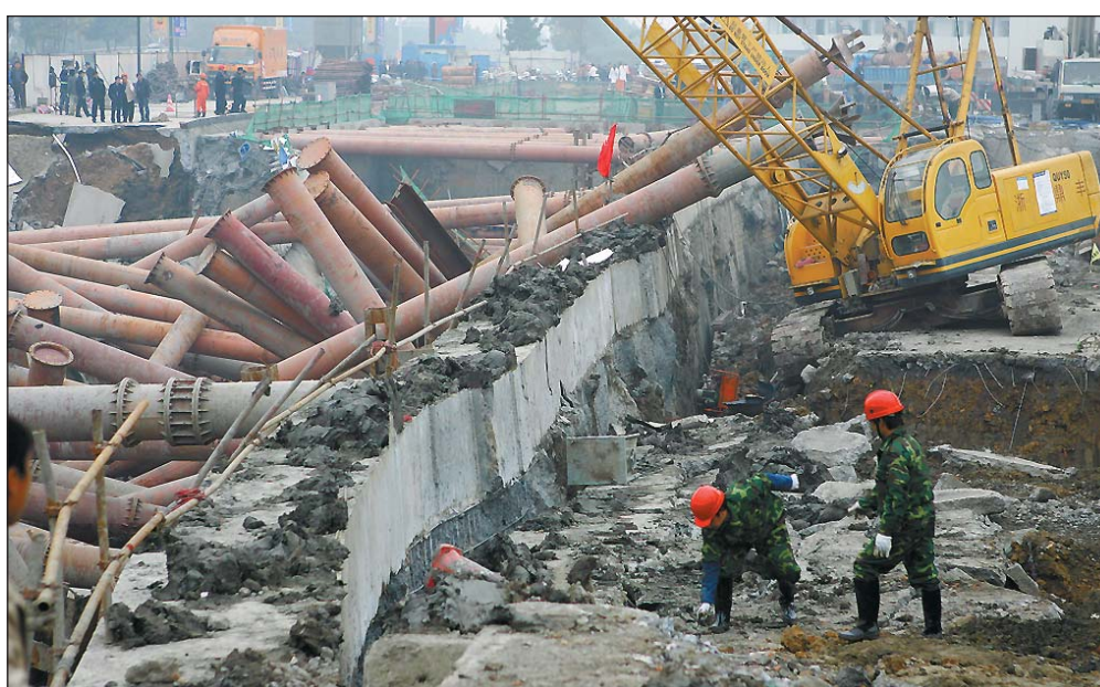
A scene of a collapse at a subway construction site that killed 21 workers in Hangzhou, Zhejiang province, in November 2008.
